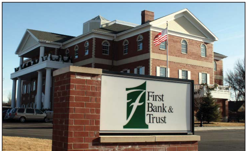
First Bank & Trust built a new downtown headquarters in Brookings in 2006.
